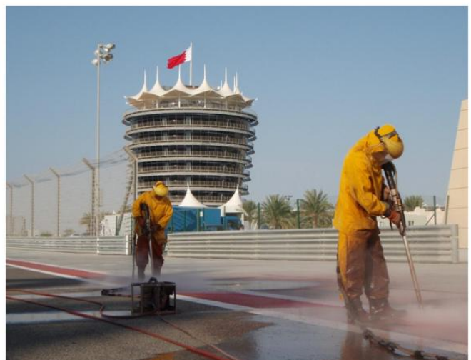
UHP water jetting, Bahrain International Circuit
