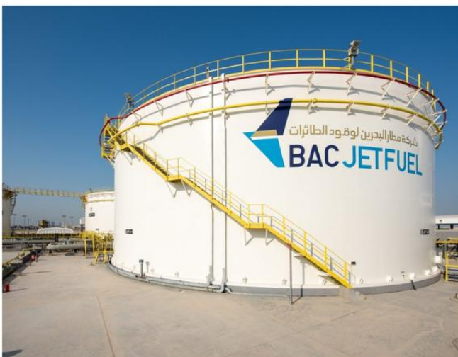
Jet fuel storage tank coating, Bahrain International Airport
